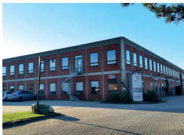
Transport-Teknik A/S, Copenhagen, Denmark
